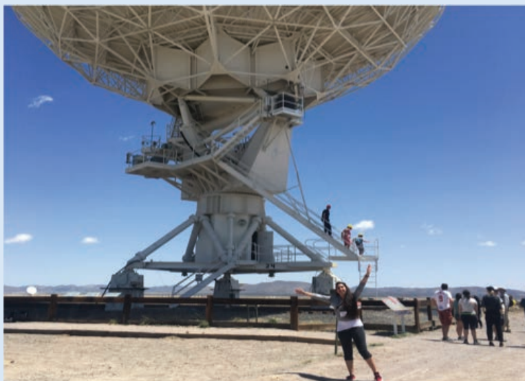
Graduate student Jessica Maldonado stands in front of a 25-meter diameter by 29-meter high radio antenna.
